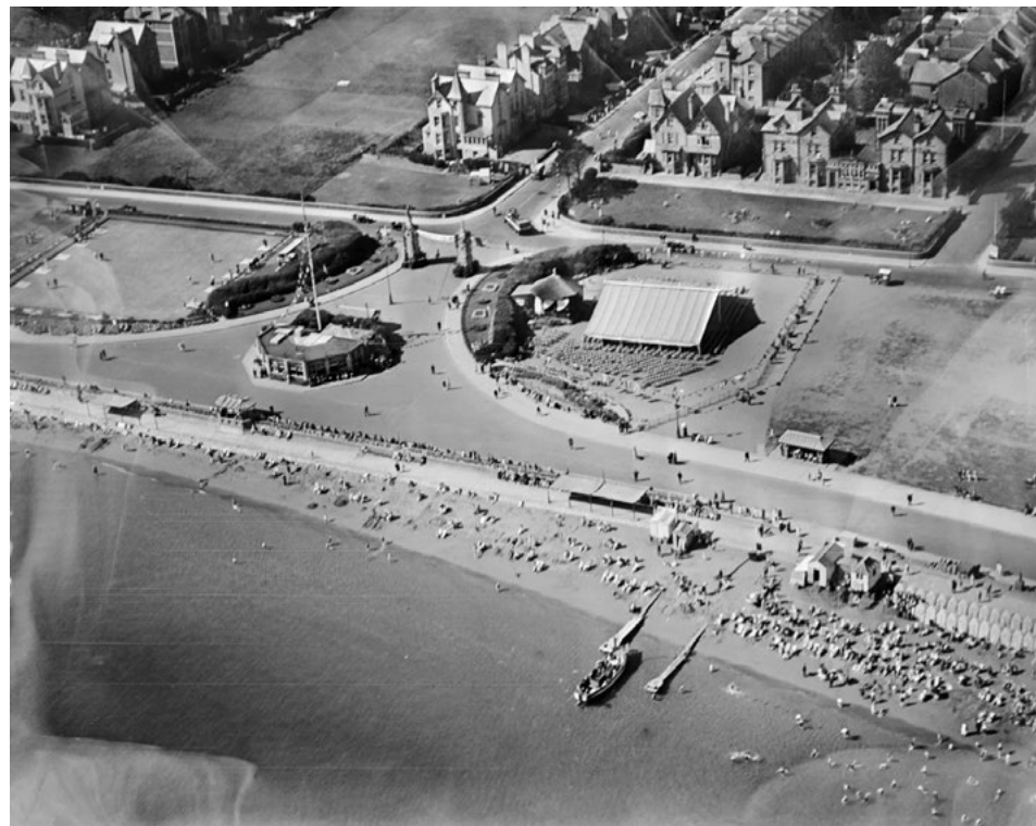
Paignton in 1928, showing an open route along Torbay Road to the sea.
